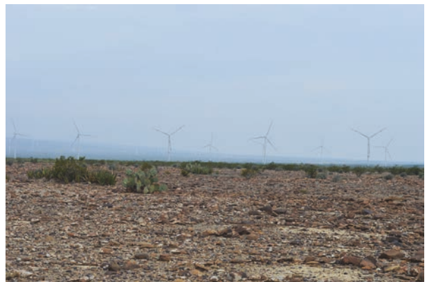
Fig. 22. Energy Projects. Wind generation of electricity near Hipolito, in the municipality of Ramos Arizpe. Photo by Manuel Nevárez de los Reyes.
